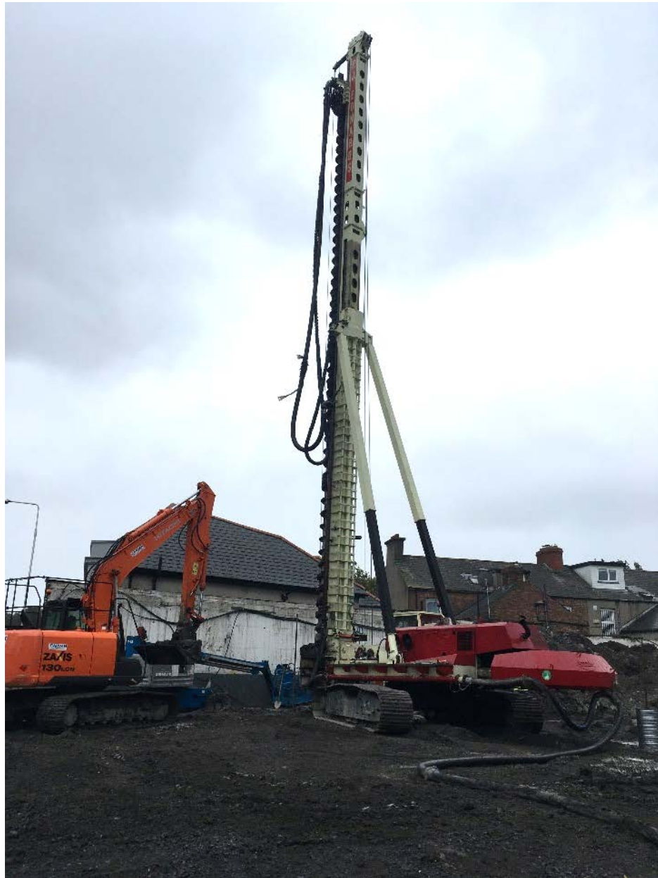
Figure 16 – Piling rig in operation
