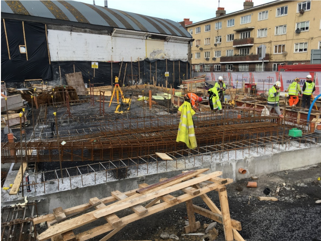
Figure 17 – Reinforced concrete ground beams cast between piles
